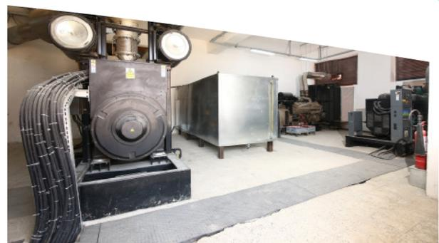
Replacing a manually run emergency power system at the Turkish Tokat Hospital, DEIF’s retrofit solution includes load sharing and returning to main power utility without interruption of power. Generators are synchronised with mains power with a smooth transfer of load to grid.
